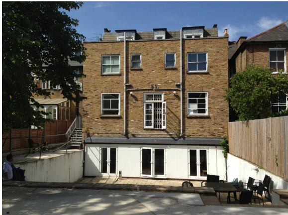
1. Photograph of existing rear elevation
