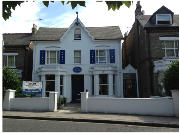
2. Photograph of existing front elevation
