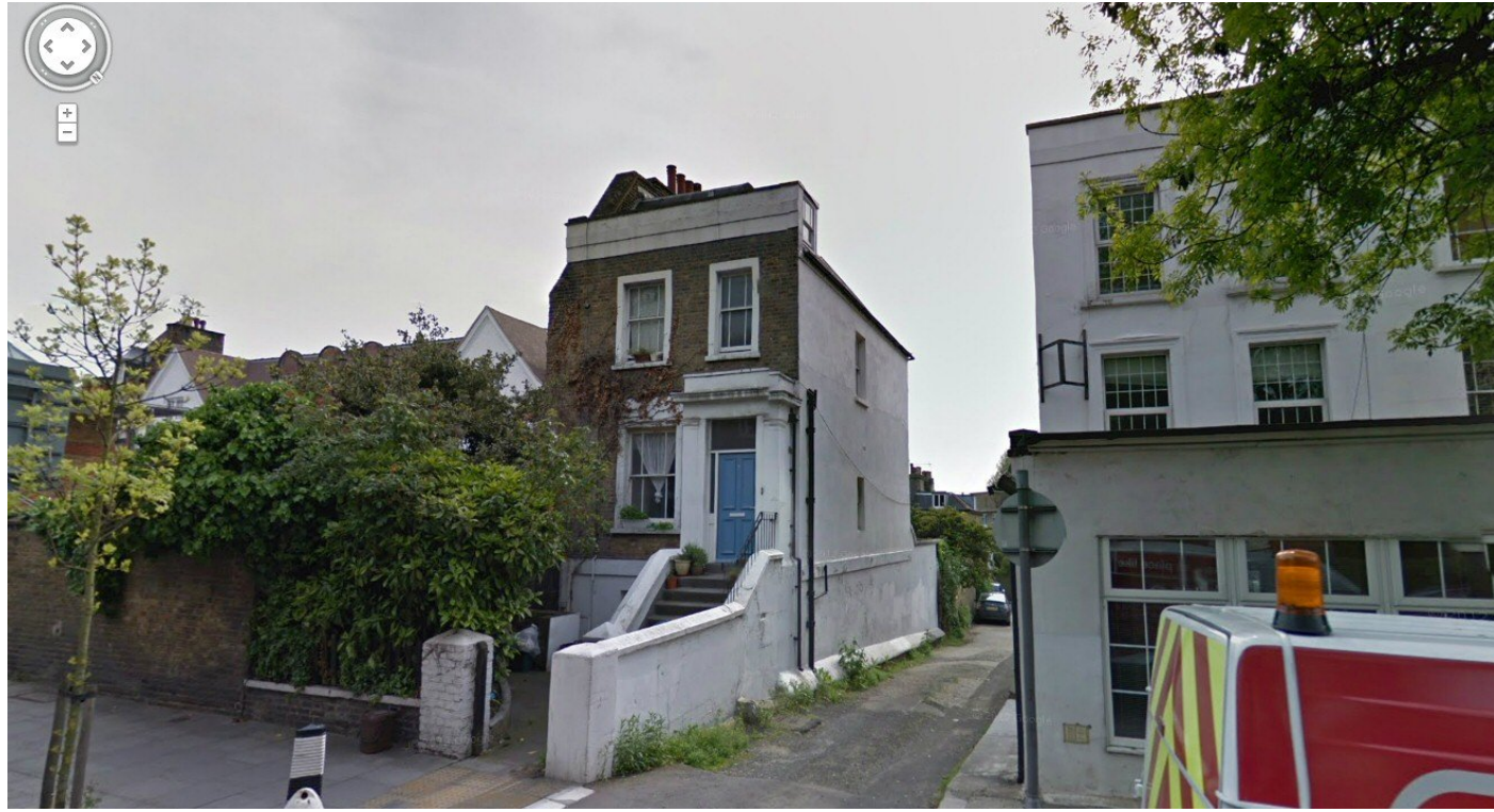
FRONT OF PROPERTY FROM TORRIANO AVENUE
