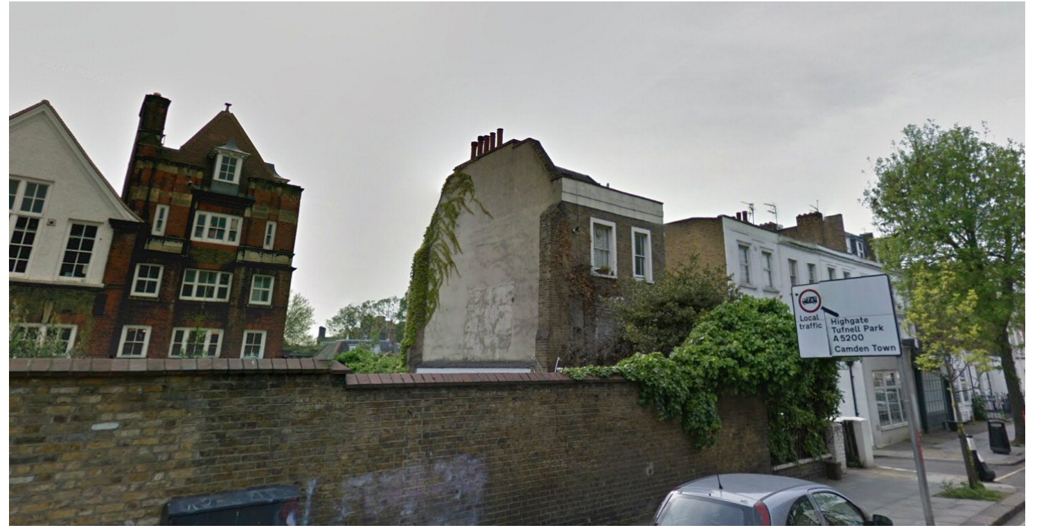
FRONT & SIDE OF PROPERTY FROM TORRIANO AVENUE
