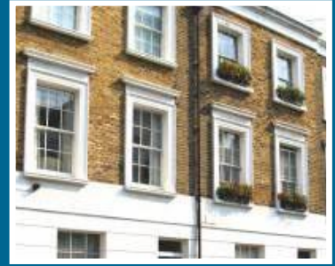
Traditional Residential Installation
