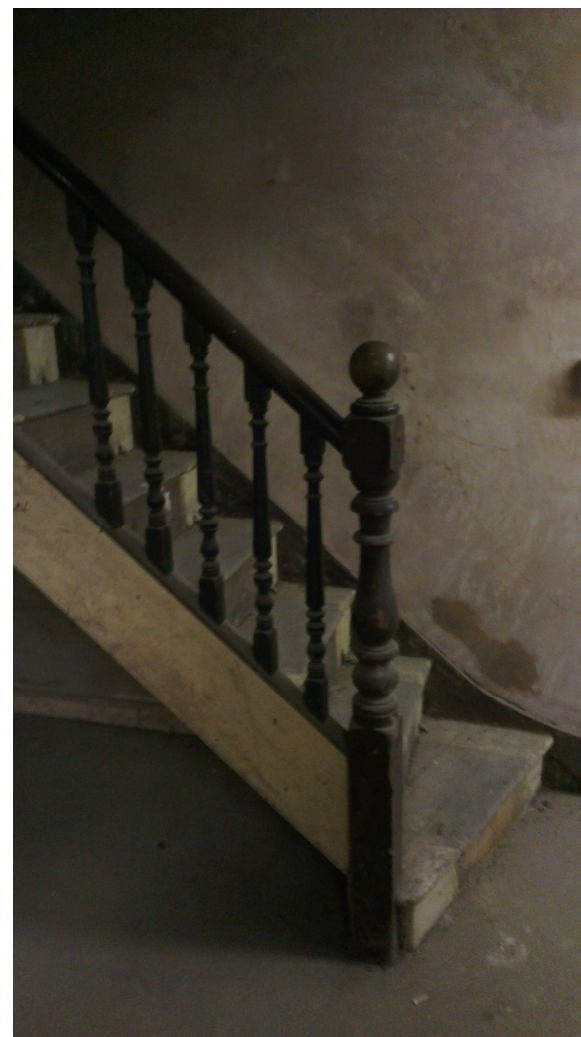
Newel post and balustrade at lower ground floor
