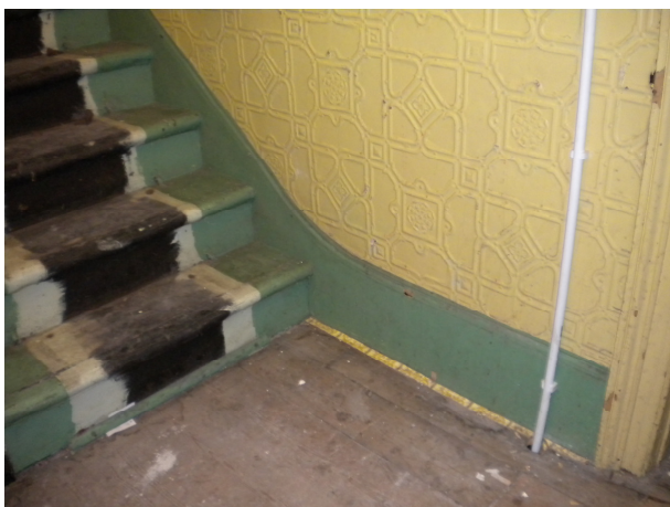
Upper ground floor bottom tread and skirting
