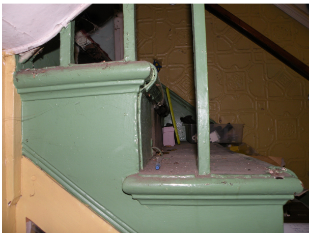
Detail of tread and skape moulding
