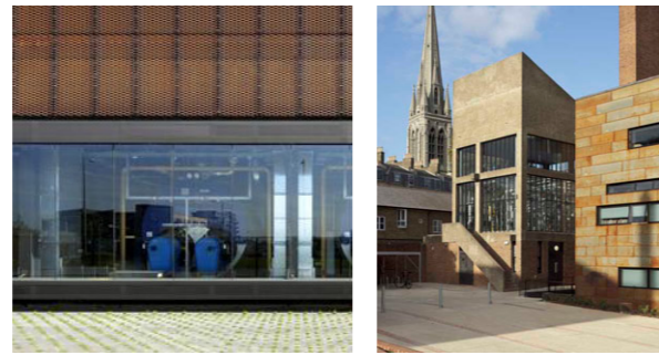
Examples of exposed plant.
