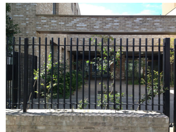
Example of a contemporary railing of a similar order to the Victorian profile version, offering good visual permeability.
