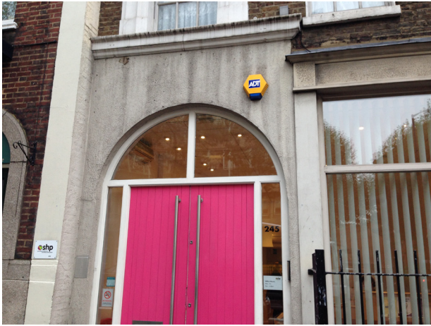
Existing office entrance doors
