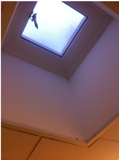
Existing small plastic rooflights
