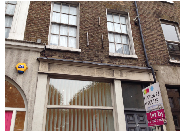
Existing clear storey glazing
