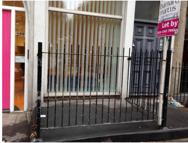
Existing reception window
