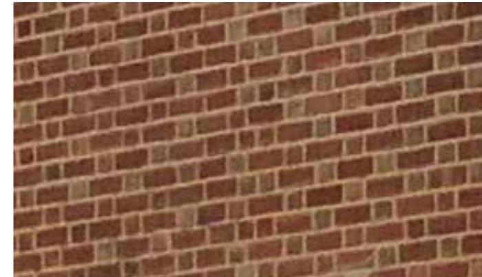
Existing bricks along Inkerman Rd
