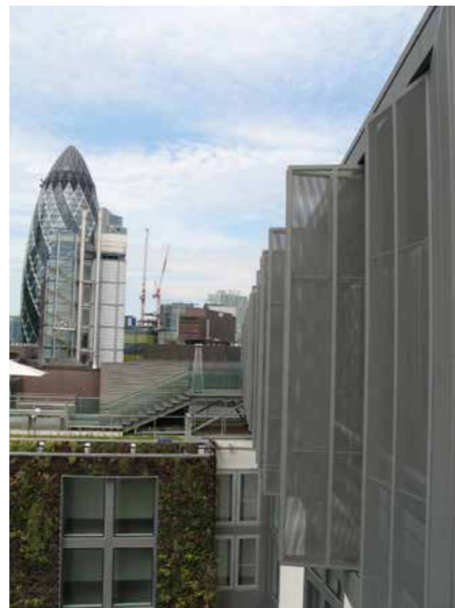
Perforated zinc shutters at the Double Tree Hotel, London.
