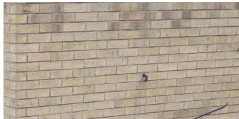
Existing brickwork to Azania Mews
