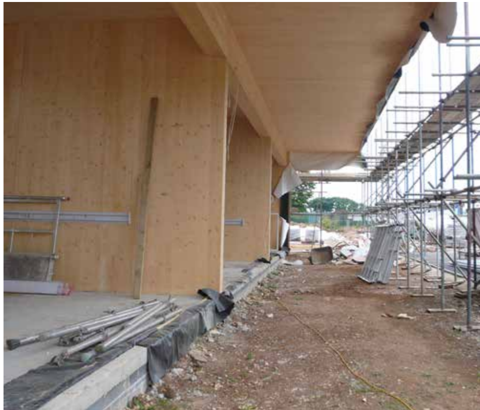
CLT walls with precut windows are erected
