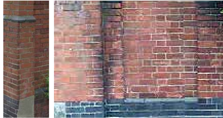
Existing brick wall to the hostel buildings
