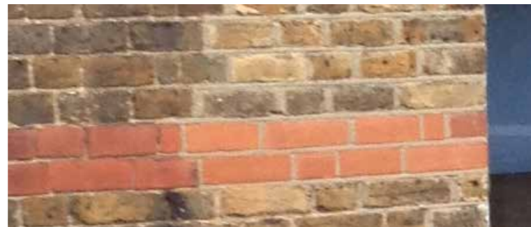
Existing brick wall to the hostel buildings
