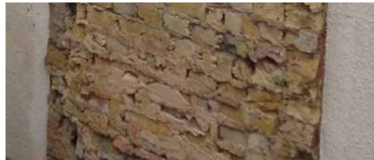
Existing brick wall to magnet superstore
