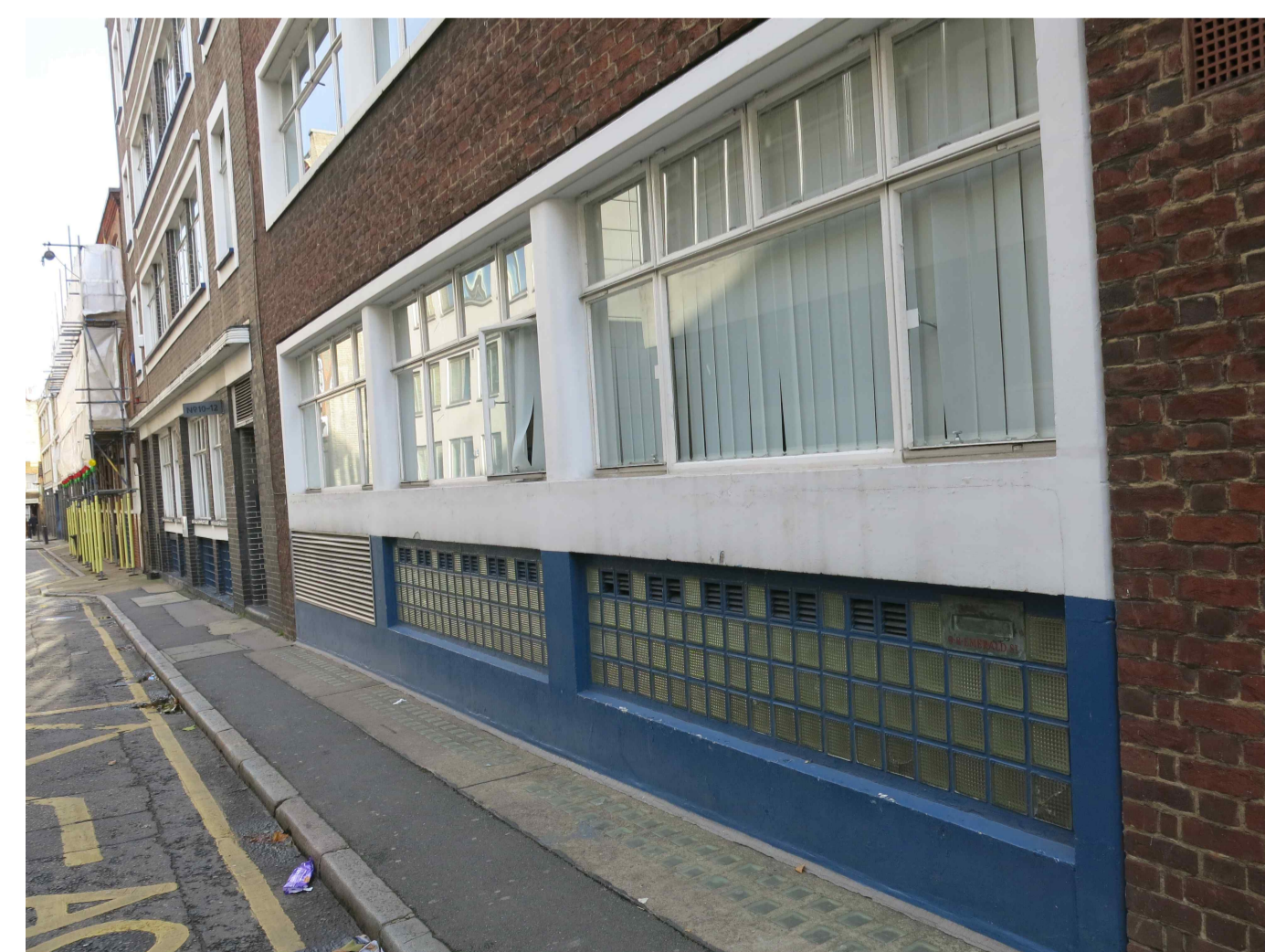
Photo showing existing facade at ground floor level
