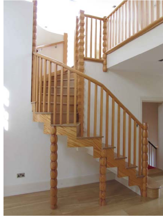
02 - Existing timber staircase
