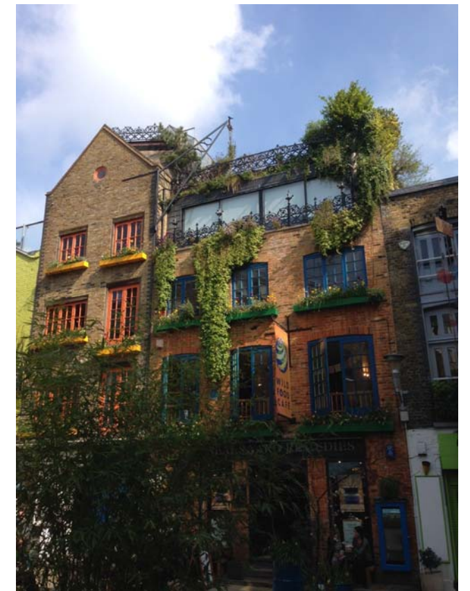
03. View within Neals Yard looking towards full width glass doors to No.14 Neals Yard.
