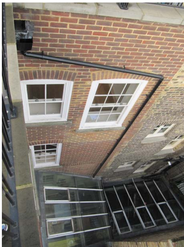
04 - Existing view from terrace to roofs below
