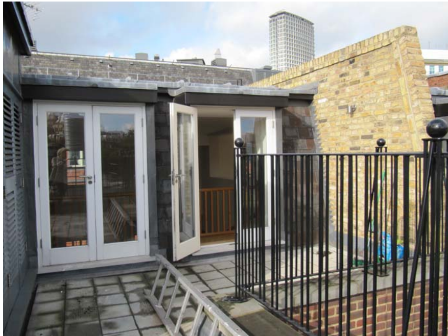
01 - Existing roof terrace with terrace doors
