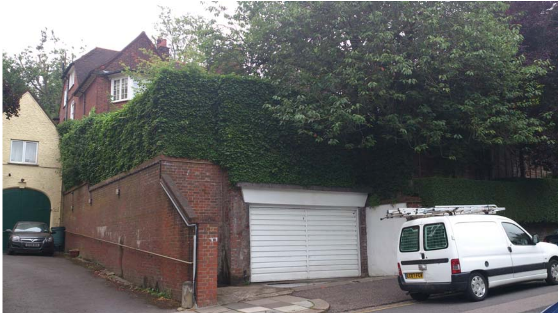
Photo 1 – Front elevation of house (behind the hedges and trees) taken from Redington Road.
