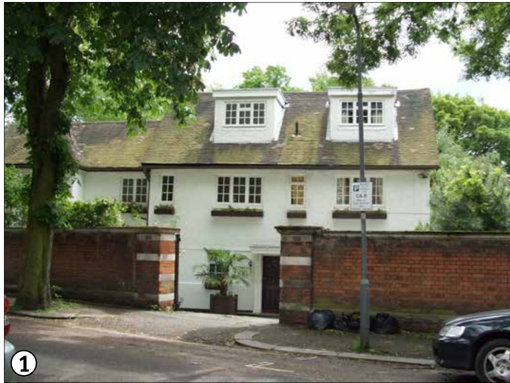
Existing house at No. 18-20 Lancaster Grove, street elevation
