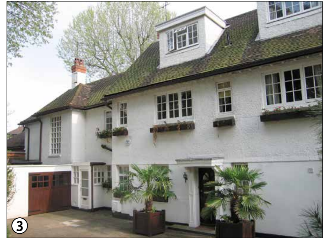
Existing house at No. 18-20 Lancaster Grove, detail of front elevation facing street. Note flat-roofed garage extension to left hand side and bulky modern dormer windows
