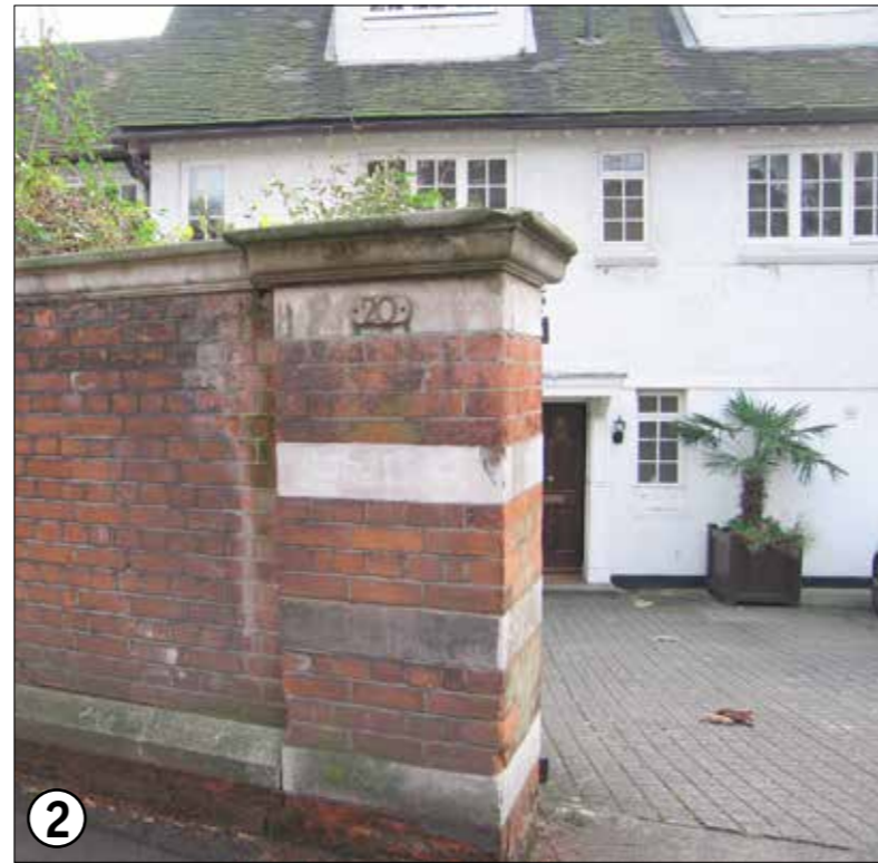
Entrance for No. 18-20 Lancaster Grove
