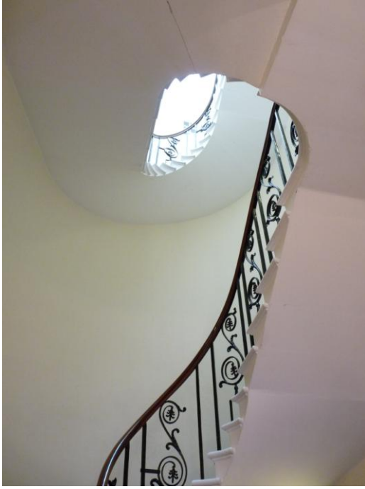
Staircases. Main staircase above. Basement staircase to left Staircase second to third floors below
