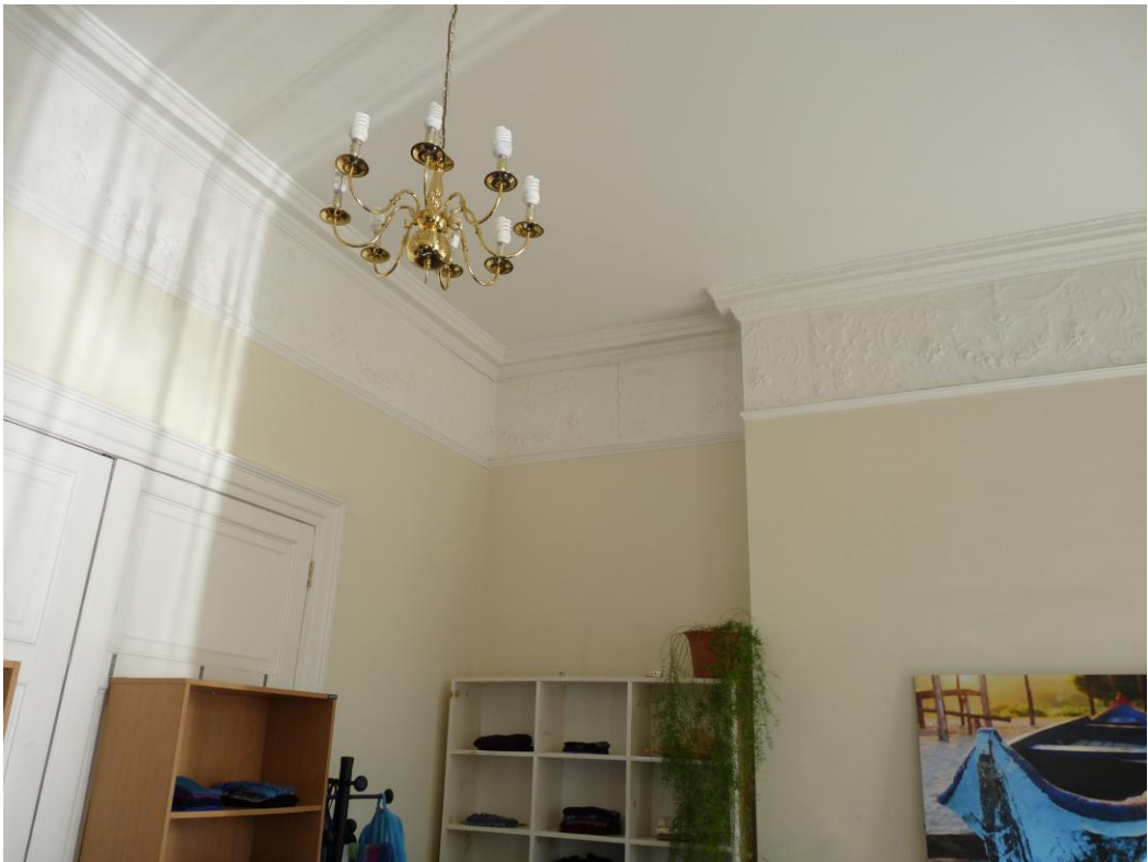
First floor principle front room
