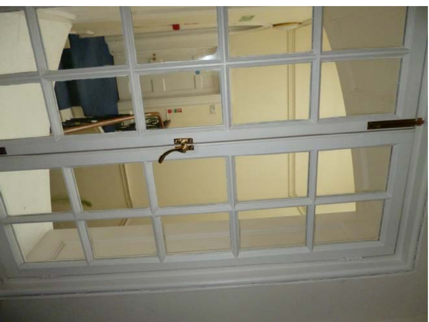
Stairwell window 2.01-x
