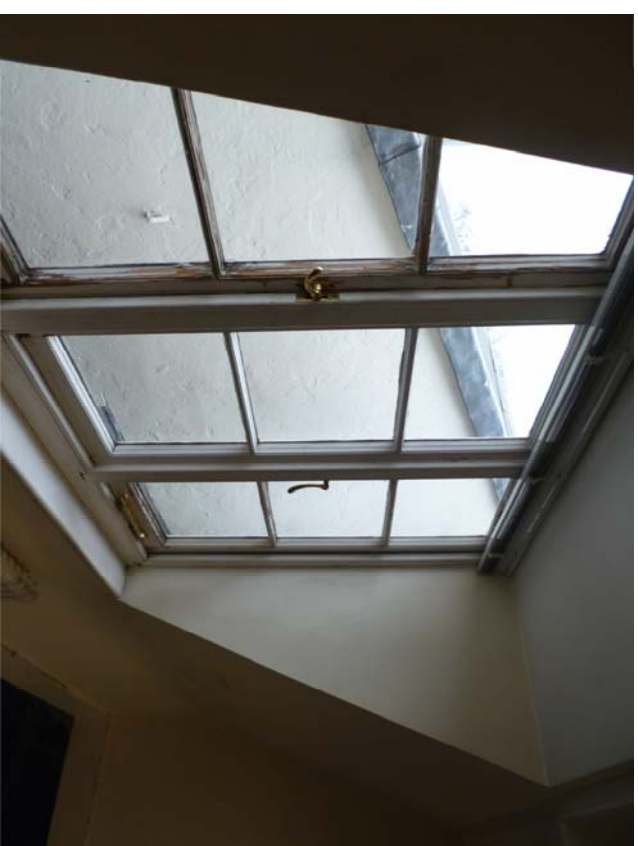
Third Floor dormer window 1.02-x
