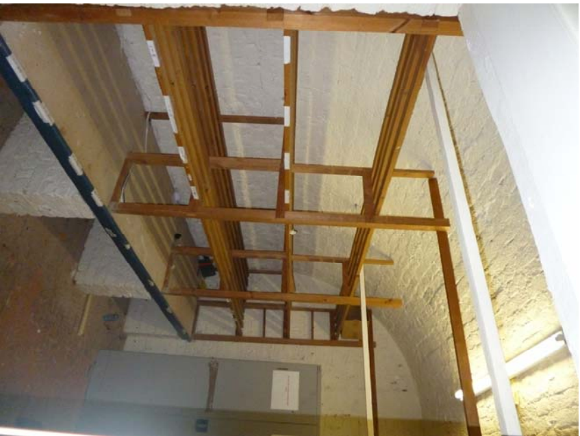
Basement vault B.05-x
