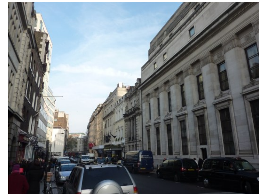
Figure 22: View from further west, with the Freemason's Hall visible on the right. The roovescape of the Kingsway Hall Hotel is more visible from this location, but is rather distant, and therefore not particularly prominent, particularly given the relative prominent and scale of other buildings, in the foreground.
