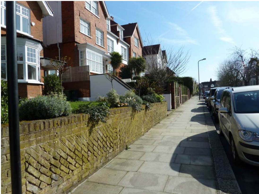
Existing brick wall of No.18 and No.16. Timber fence on No. 16.
