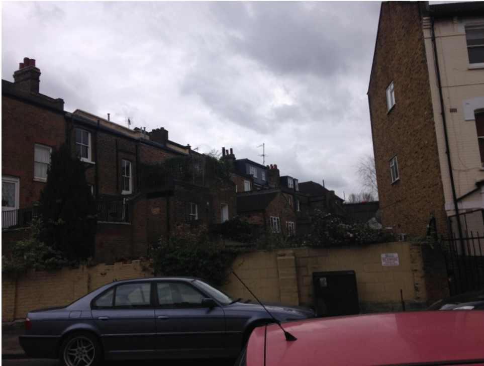
Photo 1: A view of the substantial dormer roof extensions that have been constructed in the rear roofslope of no. 3 and no. 5 Ariel Road
