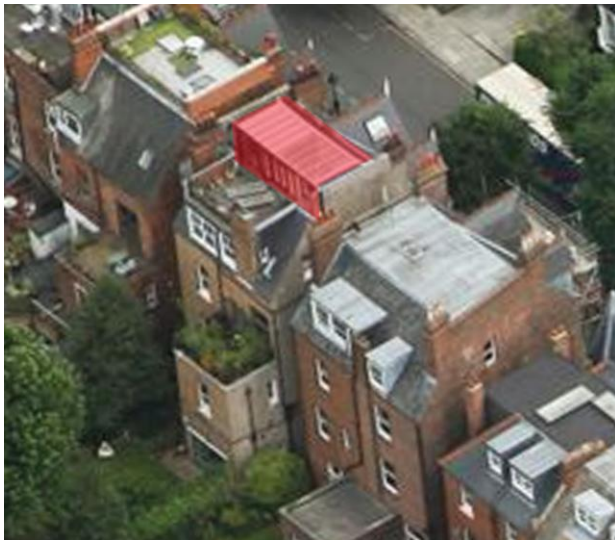
Fig. 5 - Aerial view showing roof terrace on no. 73 Parliament Hill
