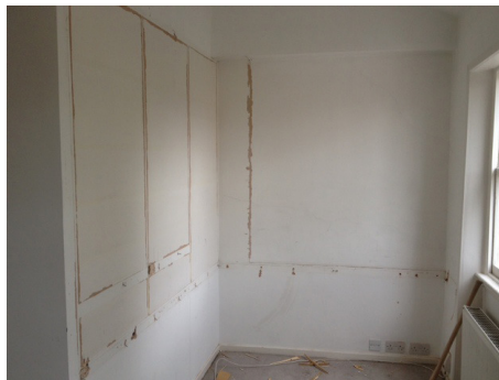
Fig 9 Third floor bathroom addition
