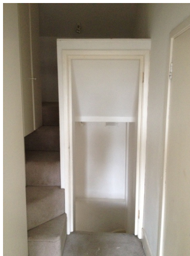
Fig 8 Upper floor staircase
