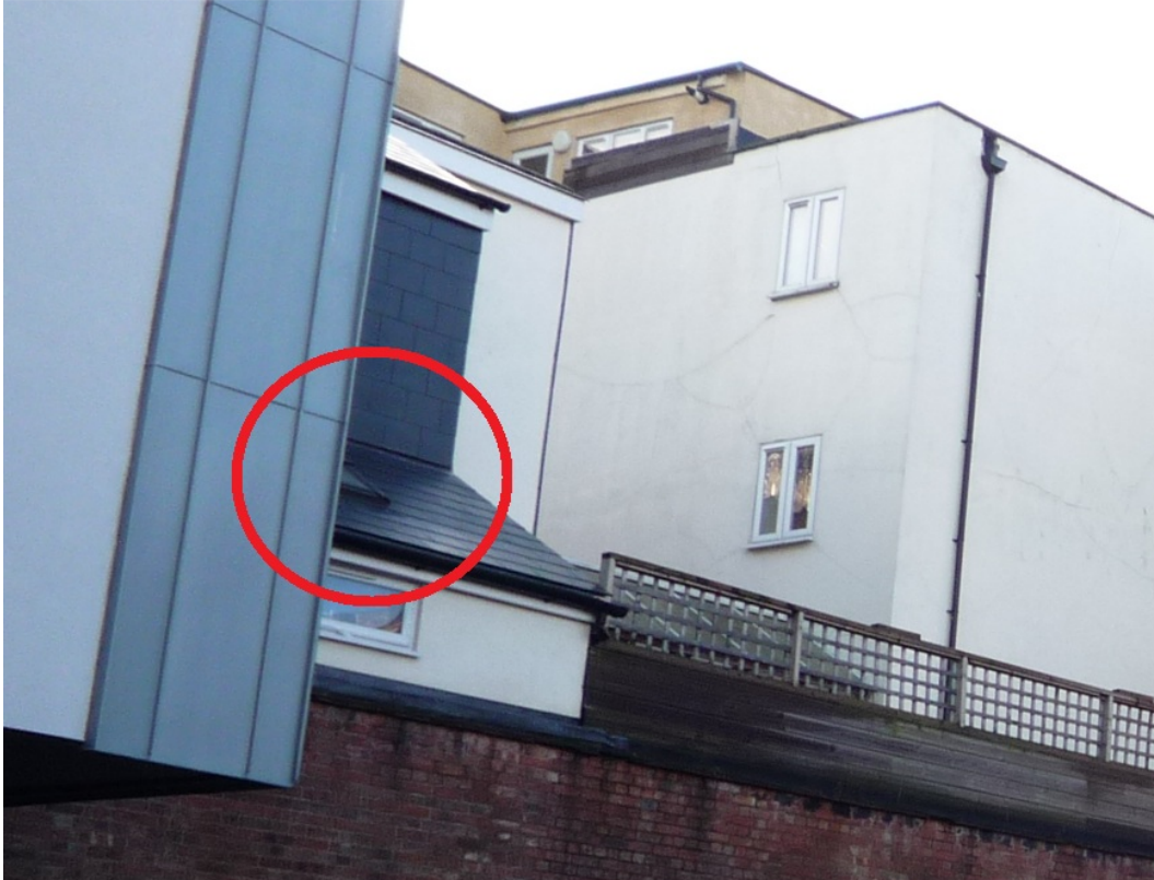
Figure 8: Skylight above Window 10
