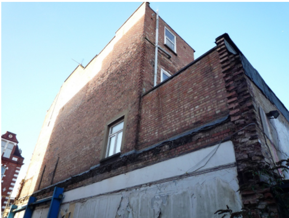
Figure 10: Existing window in flank elevation of 250 Kilburn High Road.
