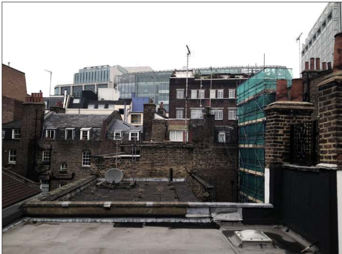
□ View from the Rooftop, looking West
