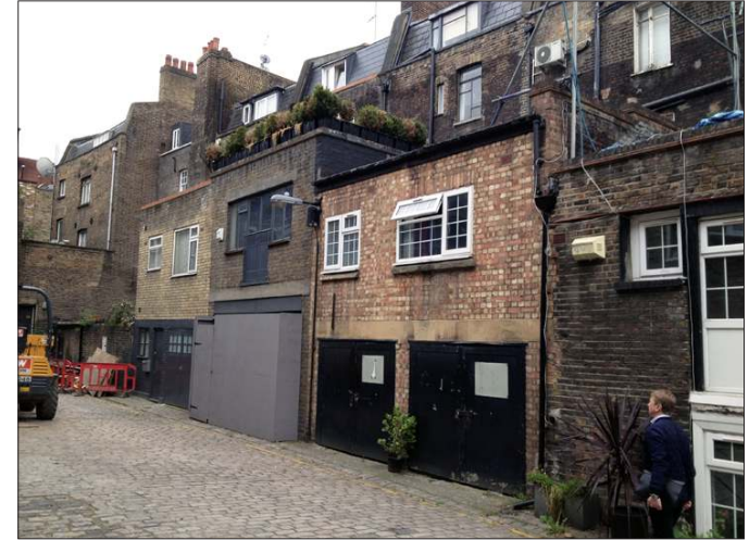
□ Rear to Cleveland Street
