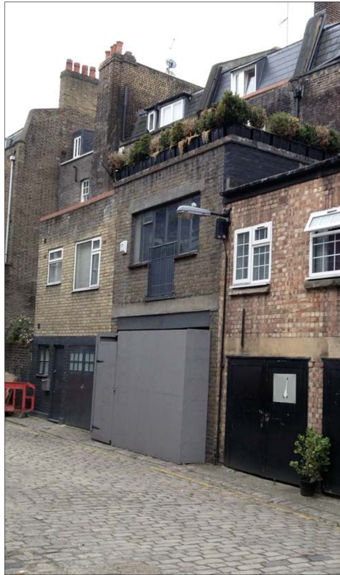
□ Existing Roof Terrace on Warren Mews
