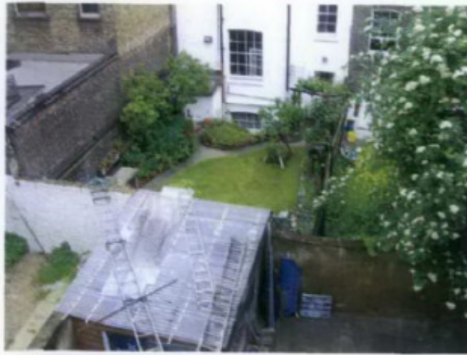
PHOTO OF ORIGINAL STORAGE SHED PRIOR TO REFURBISHMENT
