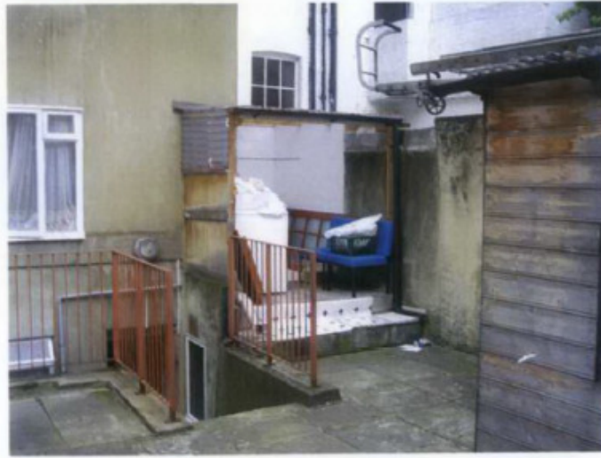
PHOTO OF SINGLE STOREY REAR EXTENSION PRIOR TO DEMOLITION
