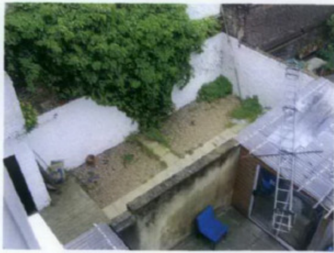
PHOTO OF ORIGINAL STORAGE SHED PRIOR TO REFURBISHMENT
