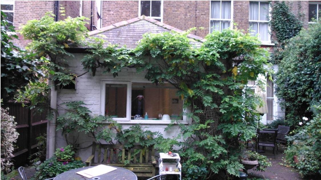
Existing Rear Extension
