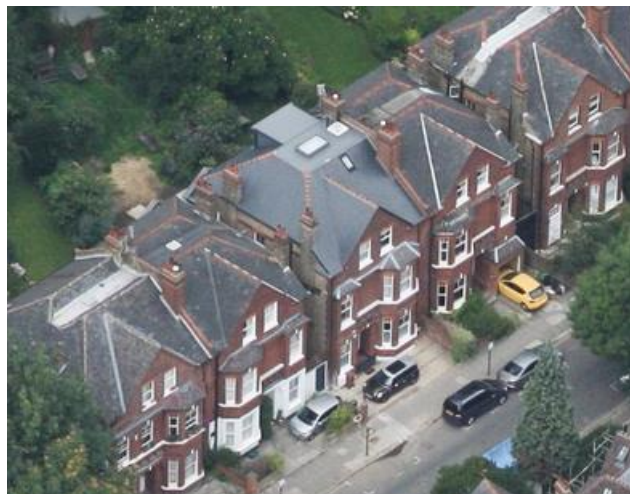
Aerial View showing similar alterations completed to No. 5 Downside Crescent
