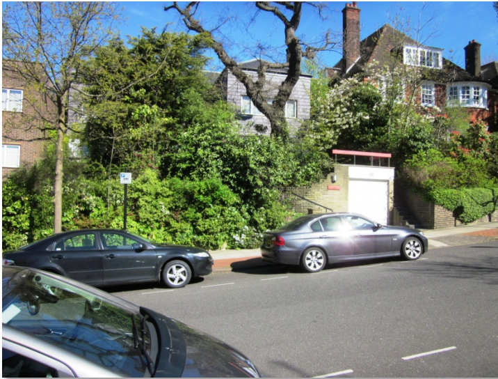
General view of the front of the property
