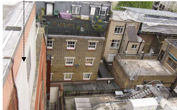
Rear plantroom wall to be replaced and extended by matching brickwork
