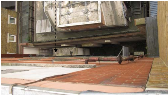
GF rear lightwell to be glazed over
