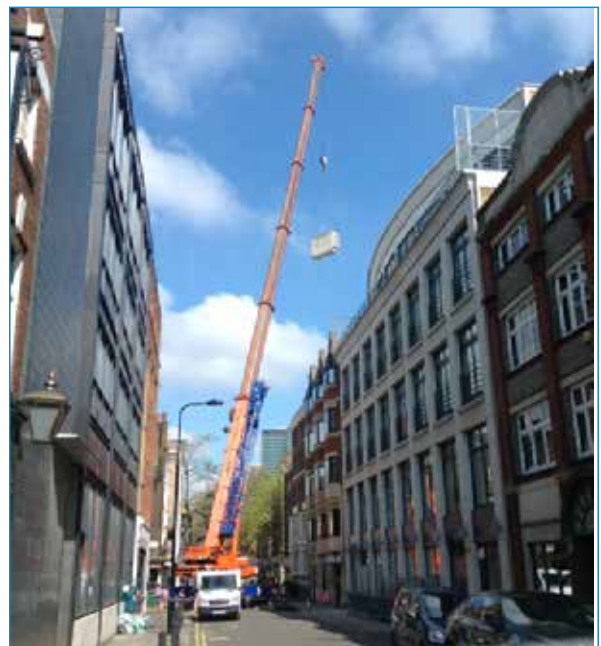
➤ Crane at Whitfield Street
