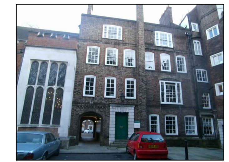
Existing and proposed elevation. Affected roof works not visible from ground level
