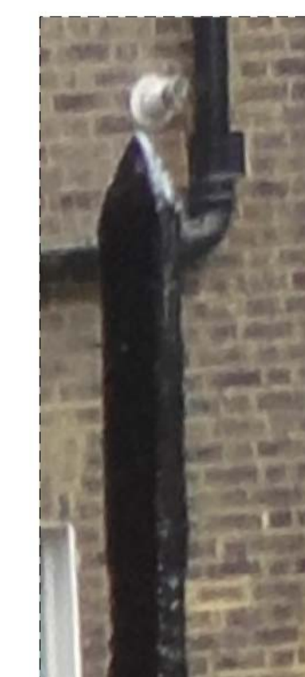
4| Image of existing Finial SLKT-1301
