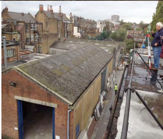
Photograph 6: An overview of the whole of the site.
