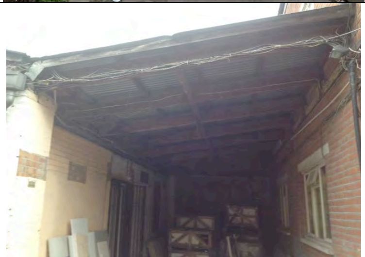
Photograph 2: One of the warehouses, note the corrugated metal roof
