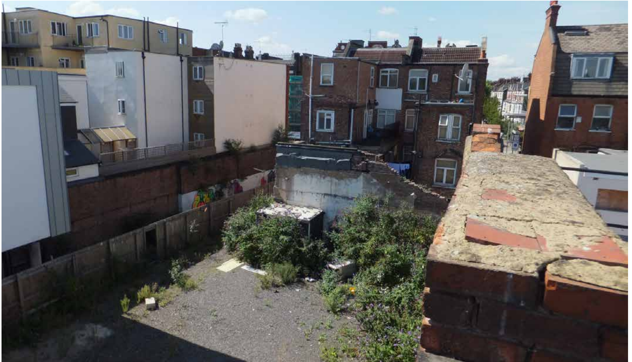
Vacant lot, with five storey development to left
