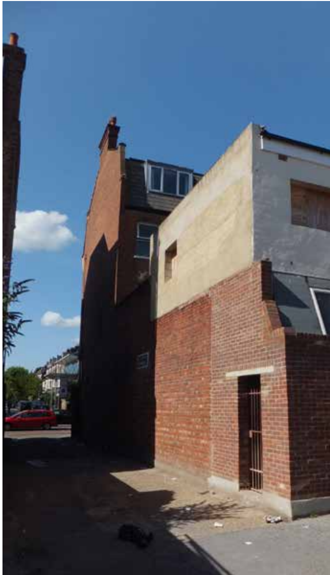
Site entrance and first floor commercial development at 252 Kilburn High Road
