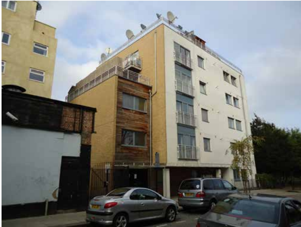
Site Photo Adjacent new build apartment block
