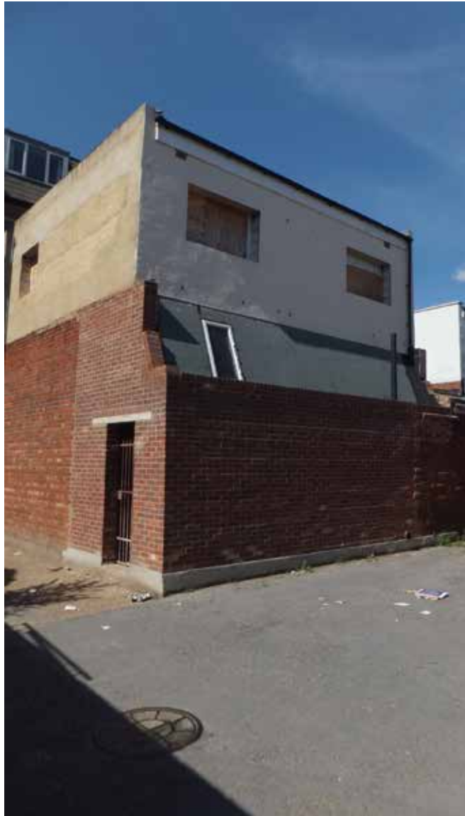
Commercial development at 252 Kilburn High Road
