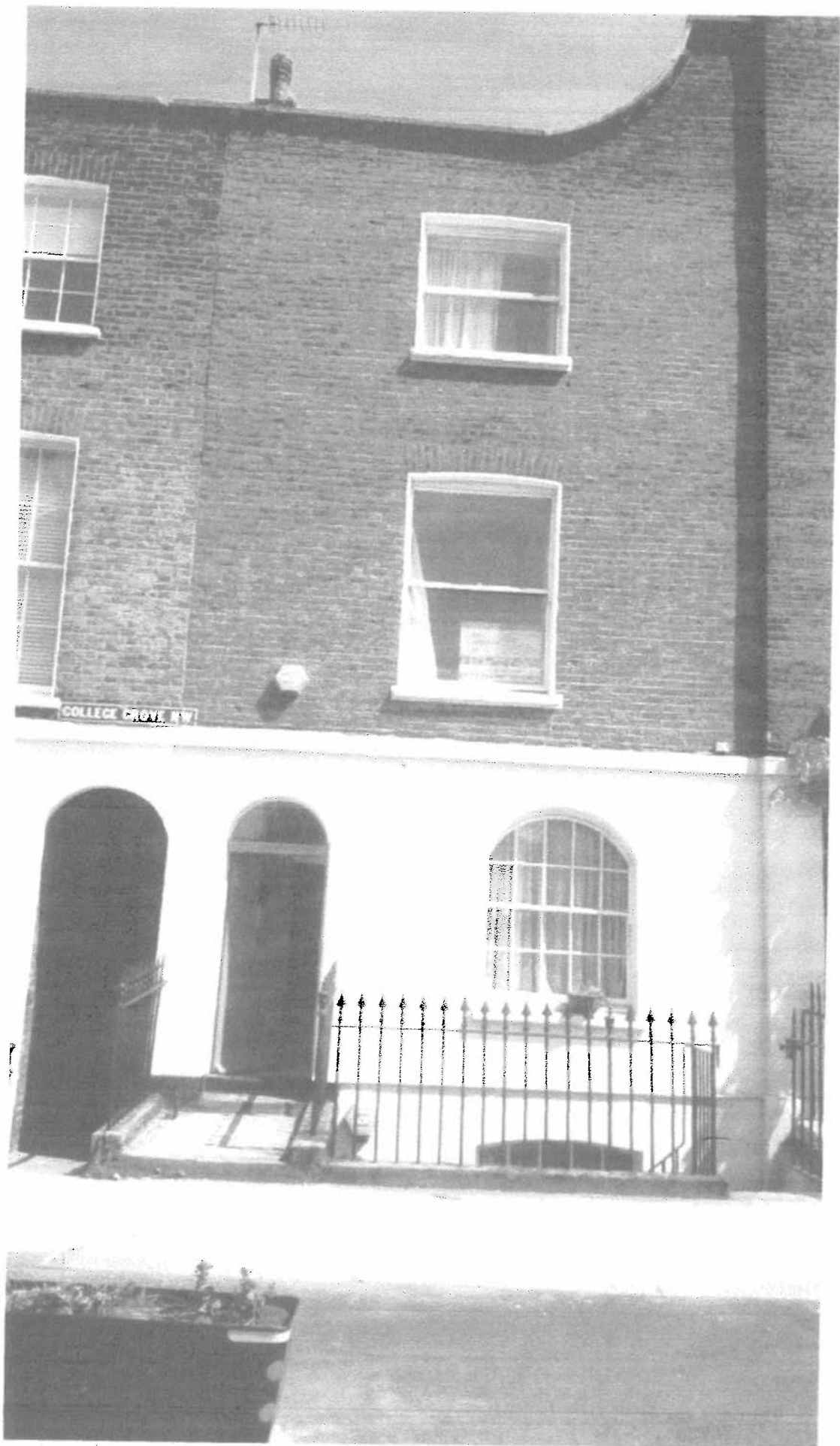
Existing Front 10 Royal College street No changes to the front
