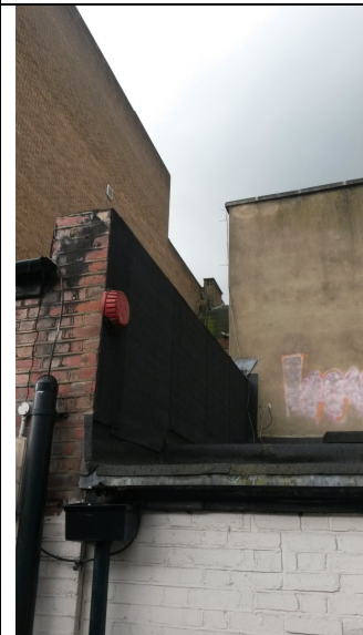
Figure 6 Flat Roofs at Rear
