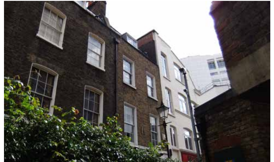
View from the garden of the Victorian terraced buildings on Tower Court
