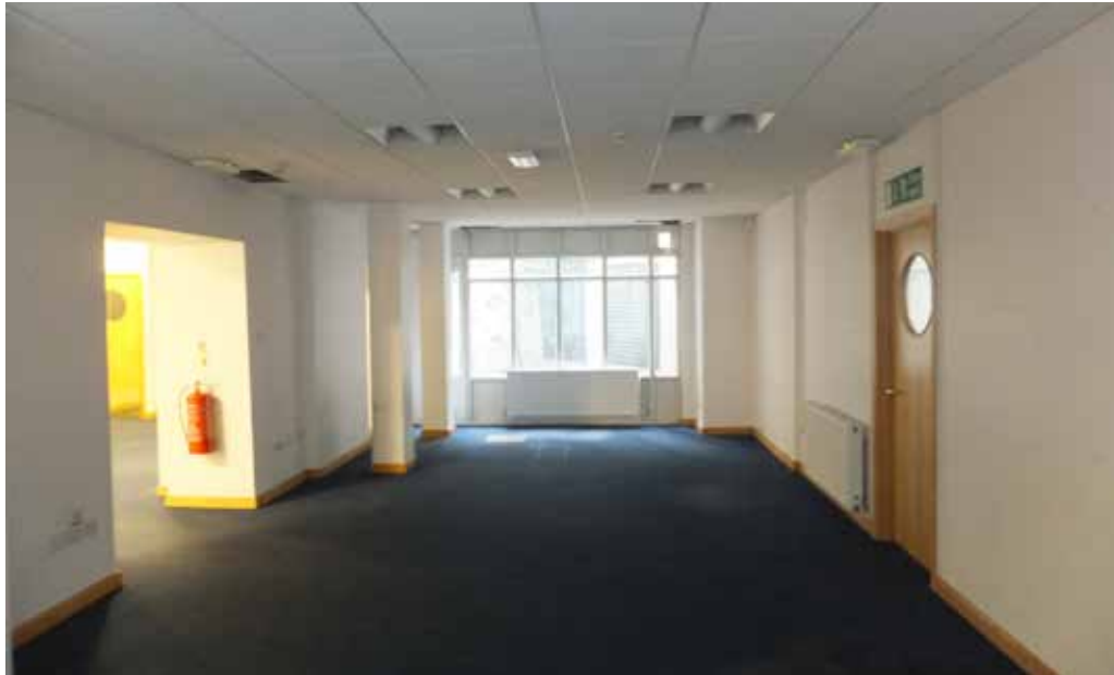
Photo of the hall area facing towards the existing light well_Corridor_Basement.
