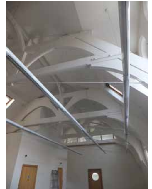
Arch Braces Trusses and their connection with the internal partitions_Fourth Floor.
