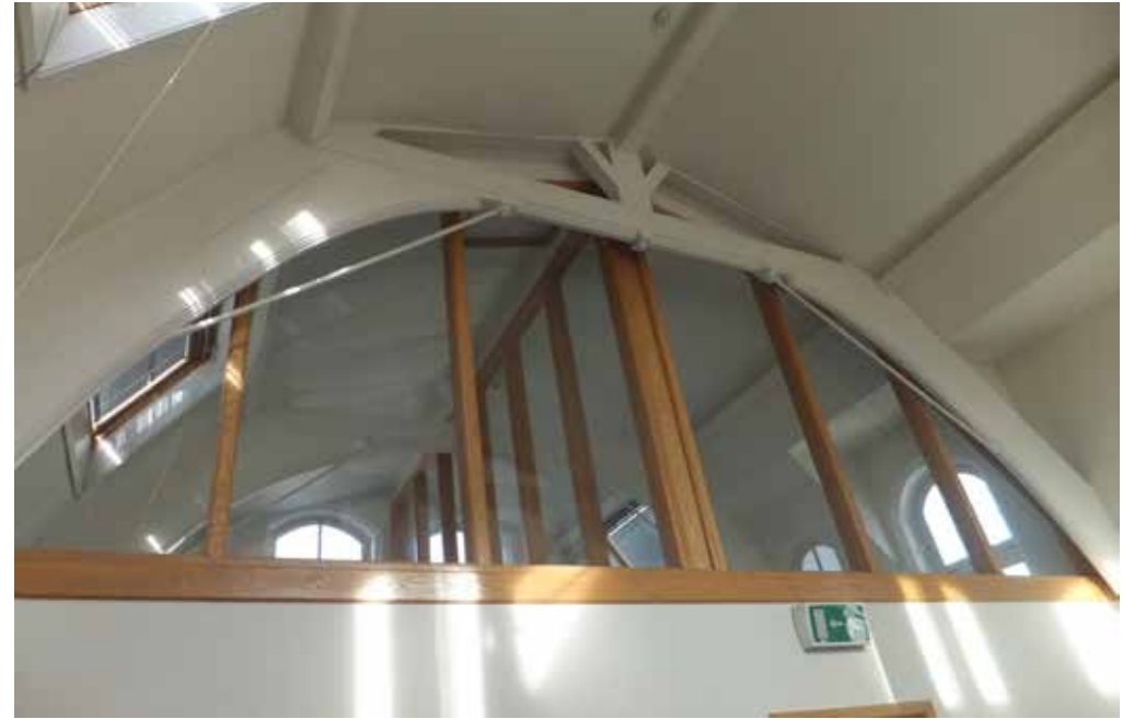
Arch Braces Trusses and their connection with the internal partitions_Fourth Floor.
