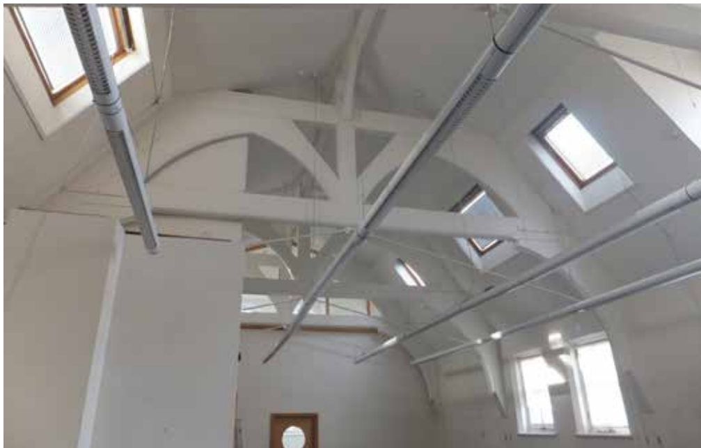
View of trusses_Fourth Floor
