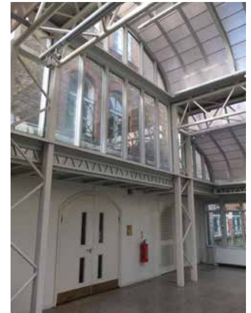
Natural lighting of both structures._Ground Floor.
