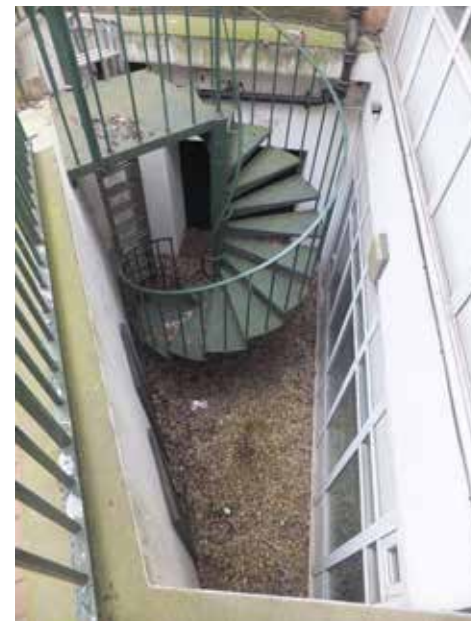
Light well_ Stair connecting basement and ground floor level.
