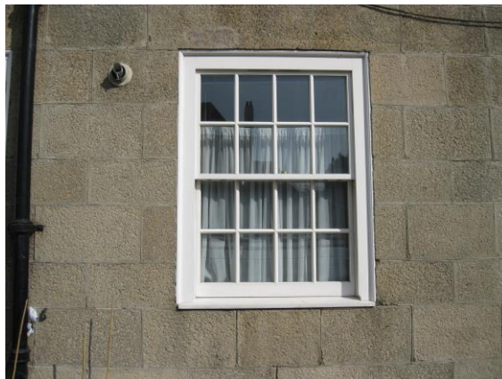
Proposed replacement timber window type as fitted in adjacent part of Levita House
