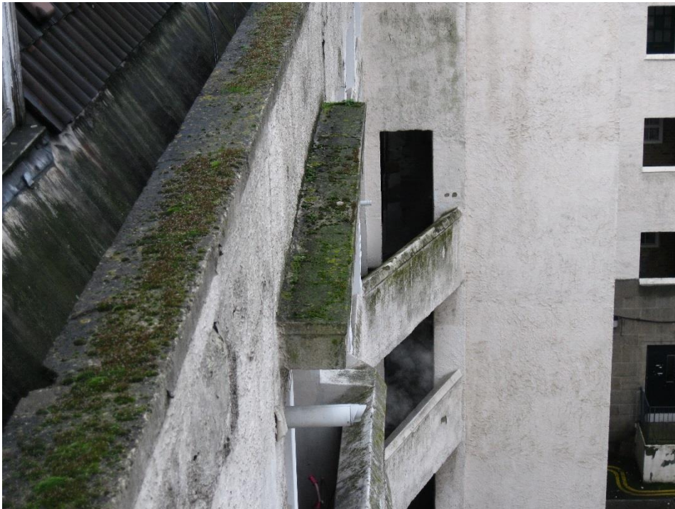
Photograph 14 Render North west side, blown
