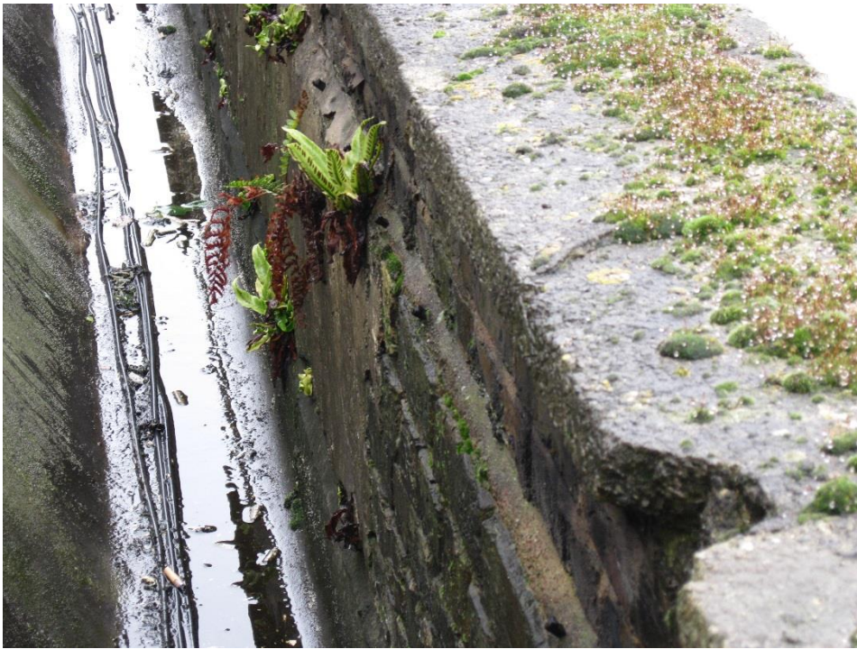
Photograph 9 Parapet wall and gutter vegetation growth
