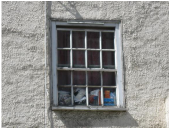
Existing sash window in 1 -21 Levita House
