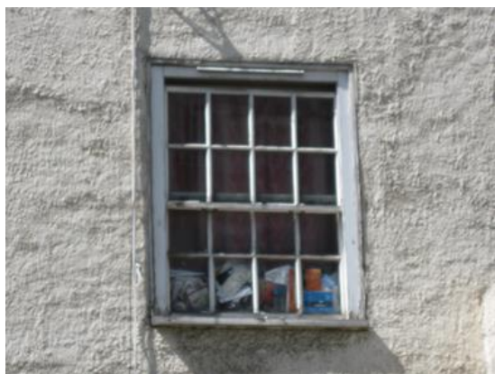
Existing sash window
