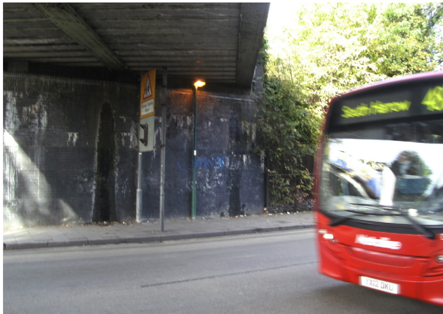
LOCATION WITHOUT POLE East side of north abutment wall of railway bridge over Acton Lane.
