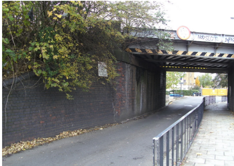
LOCATION WITHOUT POLE South abutment of railway bridge.
