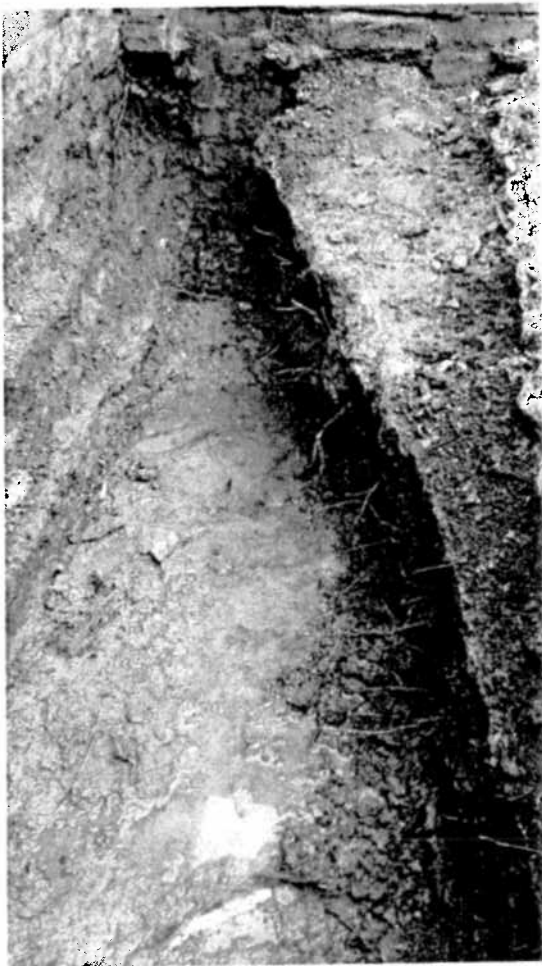
Picture 6 showing the inspection trench located parallel to the boundary wall, showing the roots from T1 – London Plane
