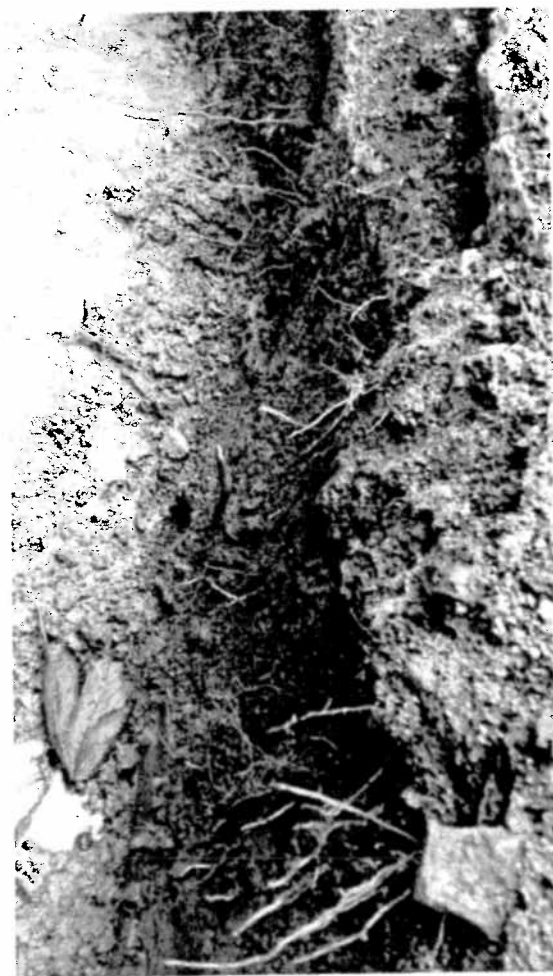
Picture 7 showing a close up of the roots encountered from T1 – London Plane, all below a diameter of 25mm
