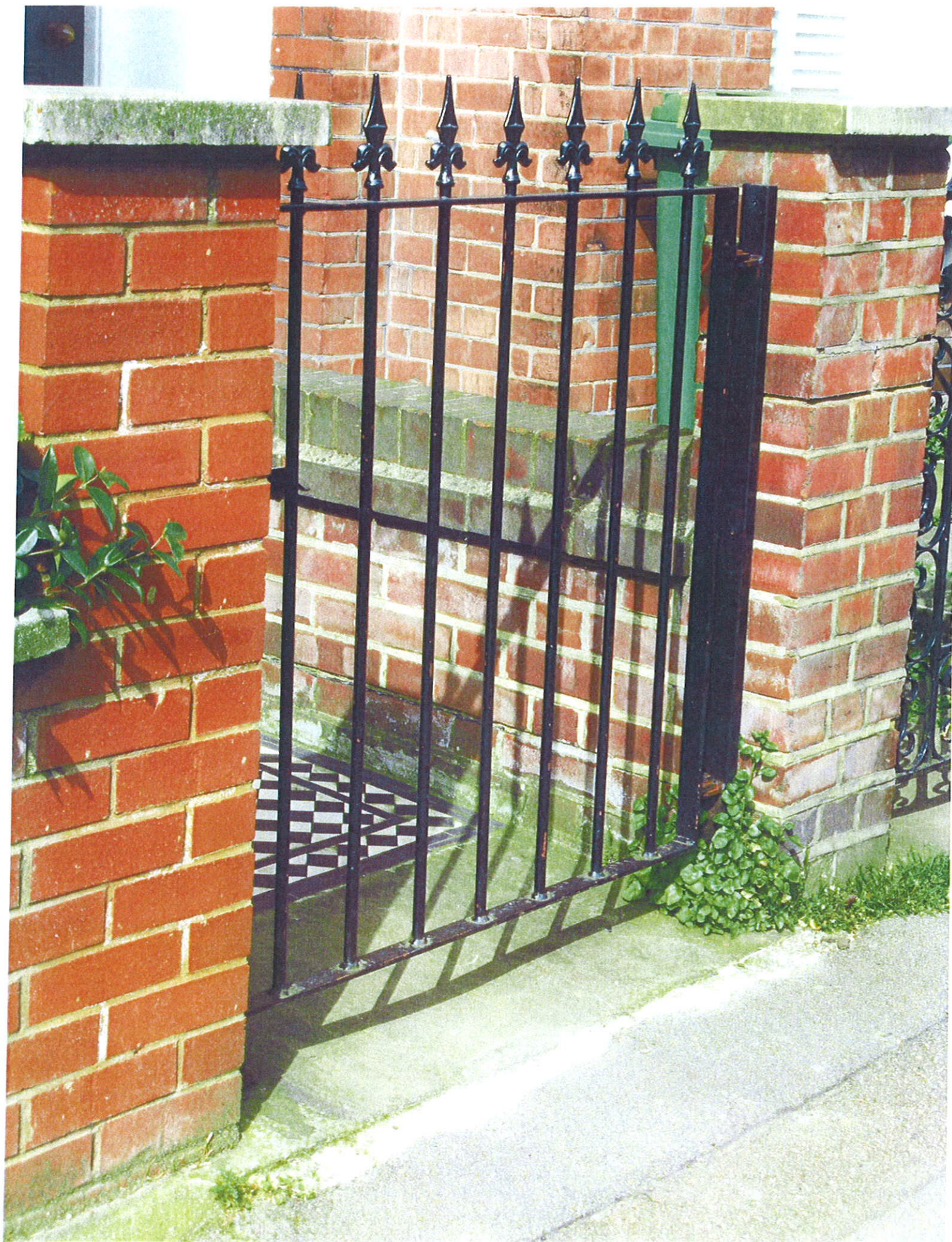
Front gate NE 13 CRESSY ROAD
