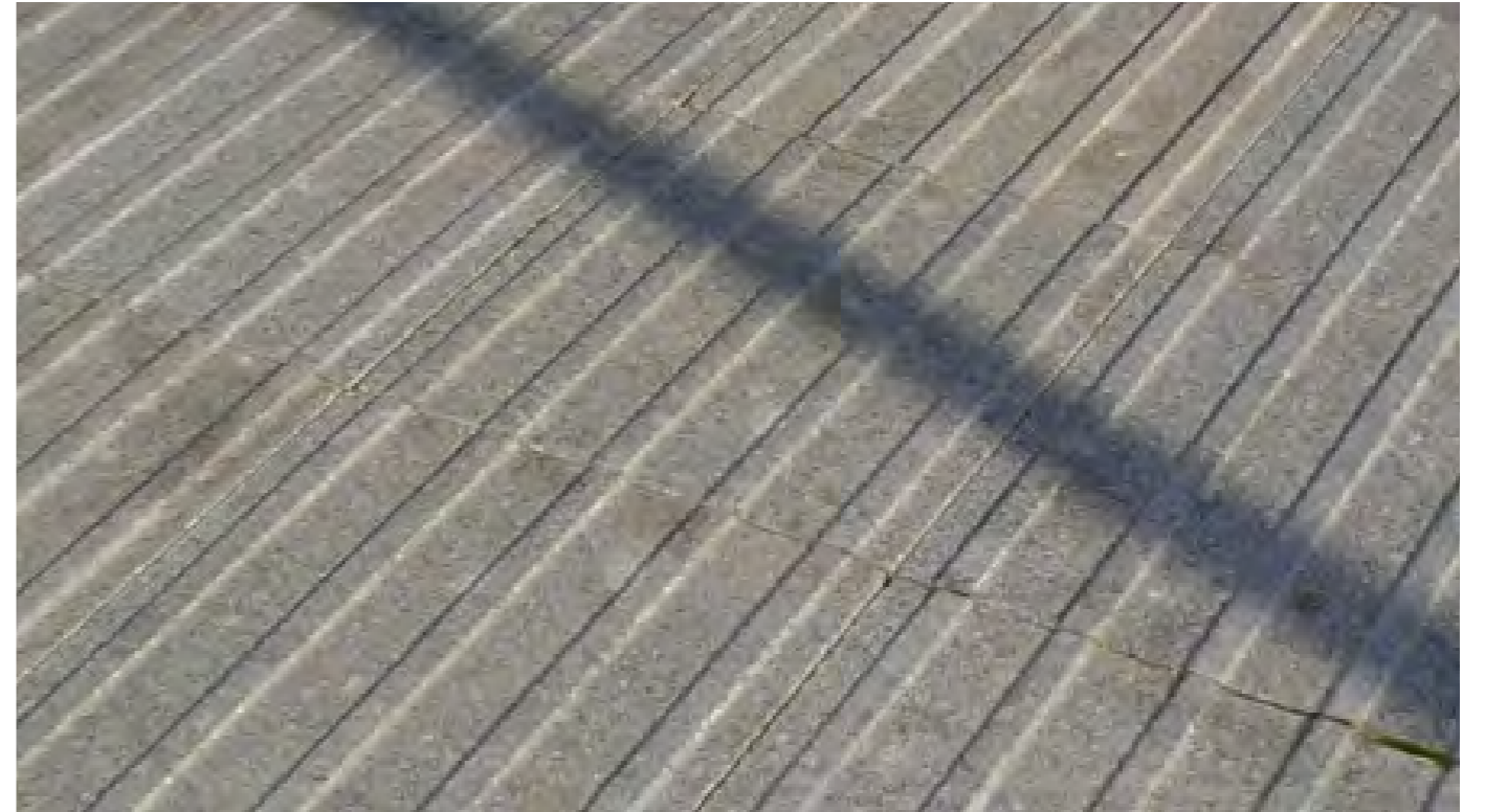
Granite Corduroy Paving
