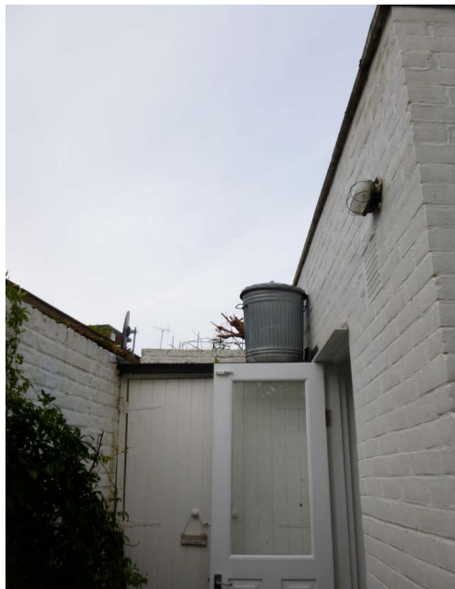
View to existing garden access and external store.
