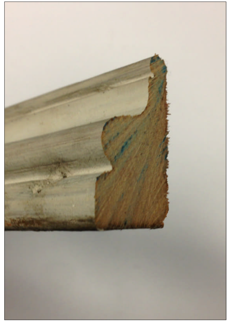
Original architrave detail from 108 St Pancras Way
