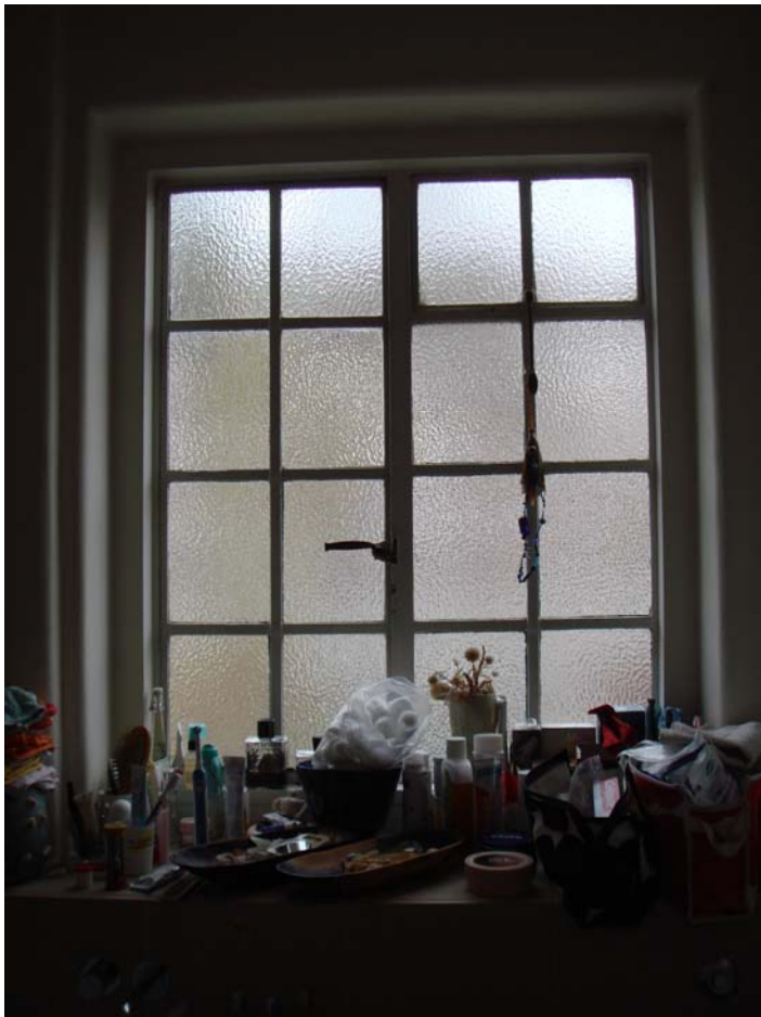
First floor (rear) crittal window to be replaced with timber sash
