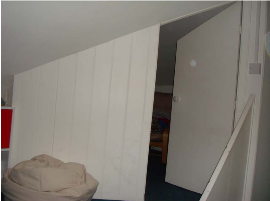
Wooden partition, door, balustrade to be removed – all later additions
