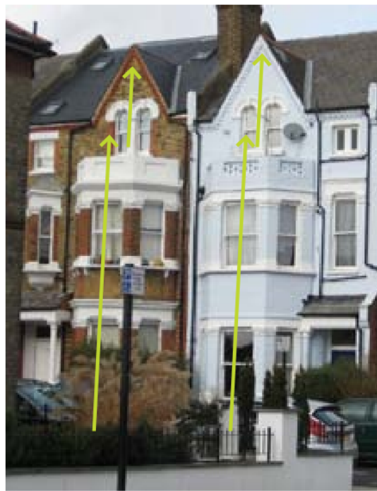
Bay windows stopping at first floor. Upper storey breaks the eaves line and animates the roof line
