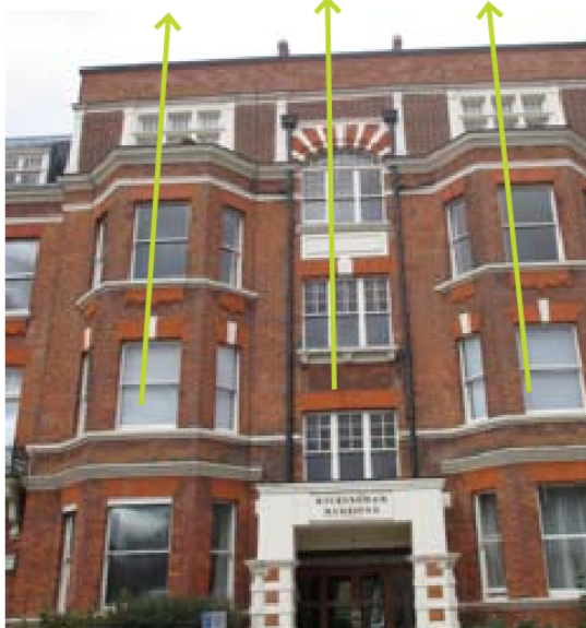
Flat roof and upper storey significantly breaking the eaves line
