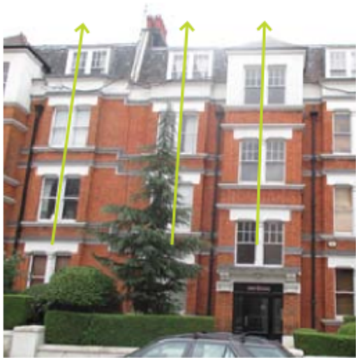
Feature Bays breaking through the eaves line
