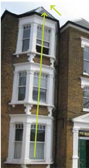
Bay windows with faceted roof capping
