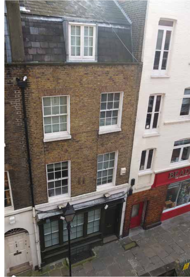
View from the upper level of the building showing one of the terraced buildings on Tower Court, highlighting the character of the Victorian street with its original street lamp.
