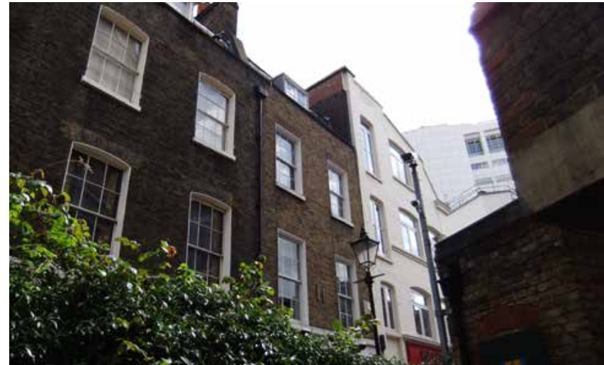
View from the garden of the Victorian terraced buildings on Tower Court
