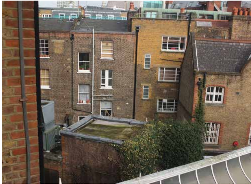
View of the rear of Earlham Street from the upper level of the building
