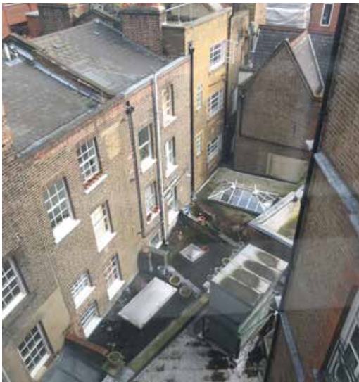
View from the upper level of the building looking at the rear of the buildings on Earlham Street.
