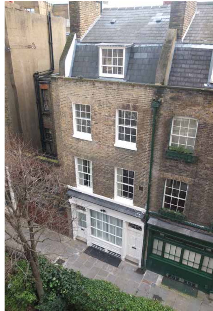
View of Victorian terraced dwelling on Tower Court Site map number _9 & _10
