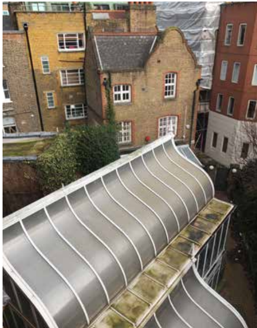
View of the rear extension looking towards Tower Court.
