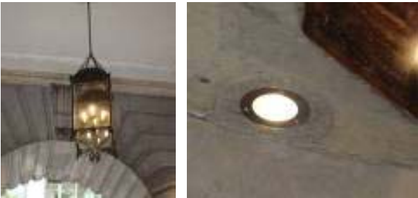
Left to right: Oversized lantern, inground uplighters.
