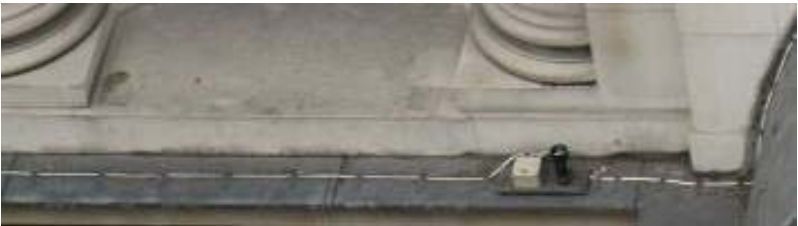
Typical installation image, i.e. cable clipped to flashing, luminaire and gear box mounted onto lead plate
