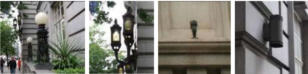
Left to right: Pedestal mounted globes, front entrance lanterns, facade uplight, low-level up/down light at base of towers
