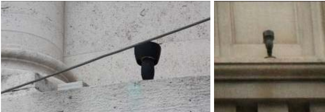
Compact spotlights onto High Holborn elevation aide visual intrusive in terms of size and scale, however, the black finish makes them visually apparent.
