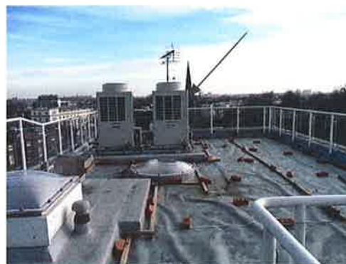
Figure 2 – 2012 Existing Condensers
