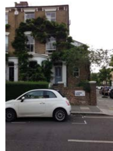
SIDE EXTENSION BUILT UP TO BOUNDARY WALL.
