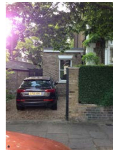
SIDE EXTENSION IN LINE WITH THE FRONT OF VICTORIAN PROPERTY, OPPOSITE 9 DARTMOUTH PARK ROAD.
