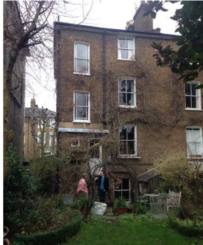
VIEW OF REAR ELEVATION OF PROPERTY
