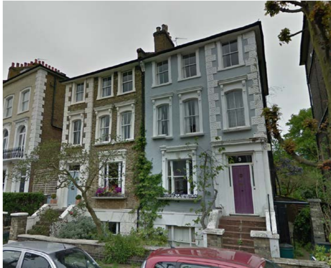
VIEW OF FRONT ELEVATION OF PROPERTY
