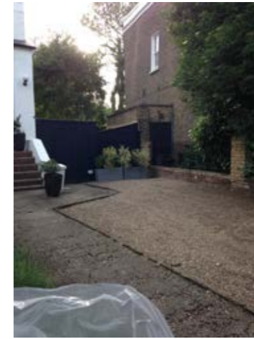
SIDE EXTENSION SET BACK, VISIBLE FROM THE STEET.
