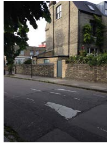
NEW LEAN-TO SIDE EXTENSION VISIBLE FROM THE STREET
