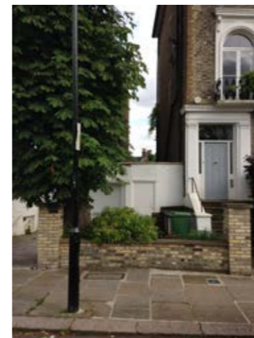
SIDE EXTENSION BUILT IN LINE WITH THE FRONT OF A PROPERTY ON DARTMOUTH PARK ROAD, OF POOR DESIGN QUALITY AND MATERIALS.
