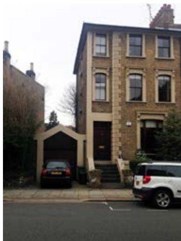
SIDE EXTENSION BUILT IN LINE WITH THE FRONT OF THE HOUSE - VISIBLE FROM THE STREET.
