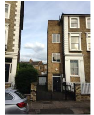
THREE STOREY SIDE EXTENSION TO A VICTORIAN PROPERTY.
