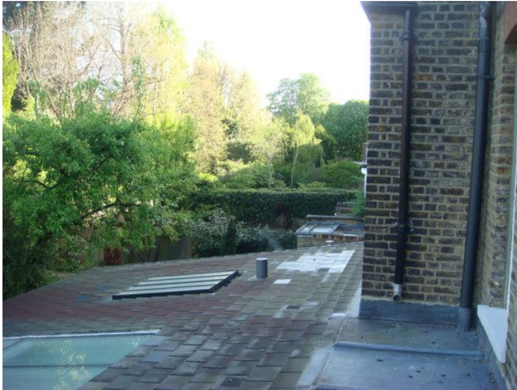
View looking towards No. 76 showing brick wall end to flat roof.
