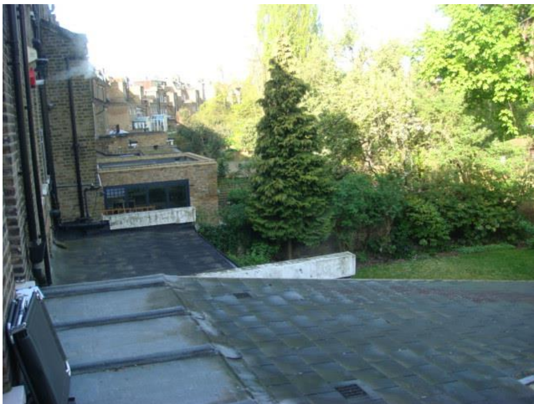
View looking towards No. 80 showing adjacent flat roof.
