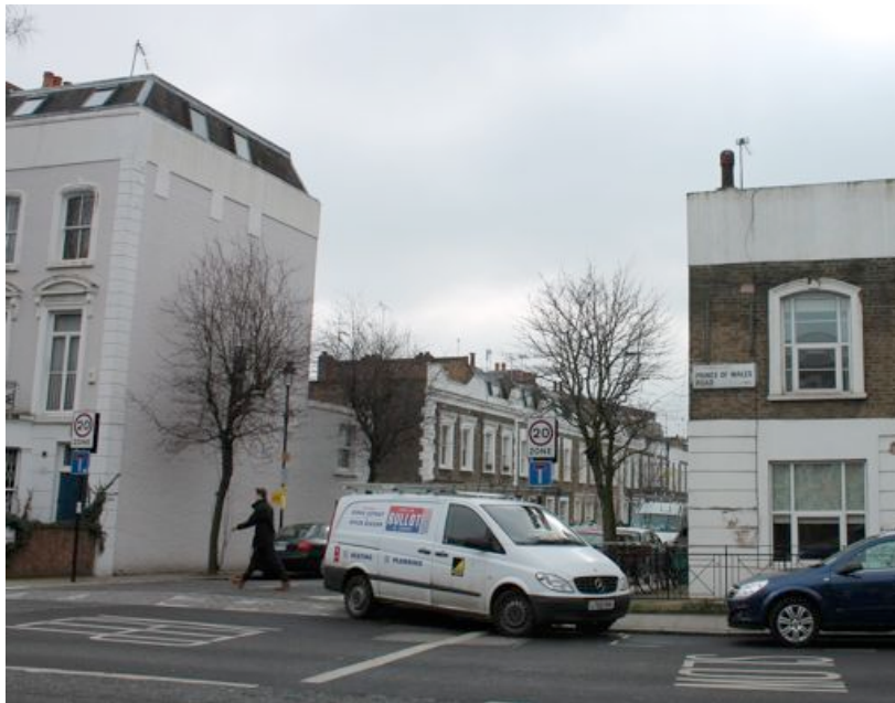
The flank wall to 49 Prince of Wales Road facing 2a Hadley Street.
